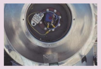
Figure 4.16 Flange side of the hot water storage tank with the electrc heater, the thermostat and the anode
