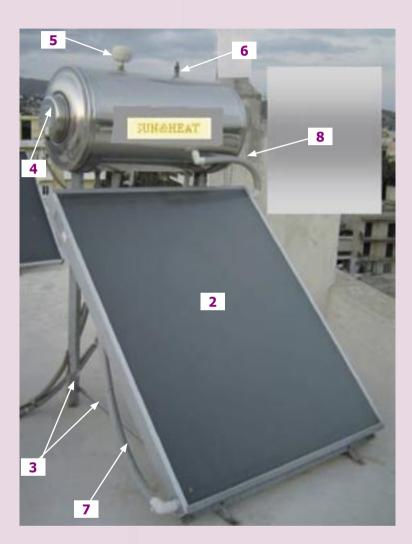
1. Hot water storage tank 2. Solar collector
