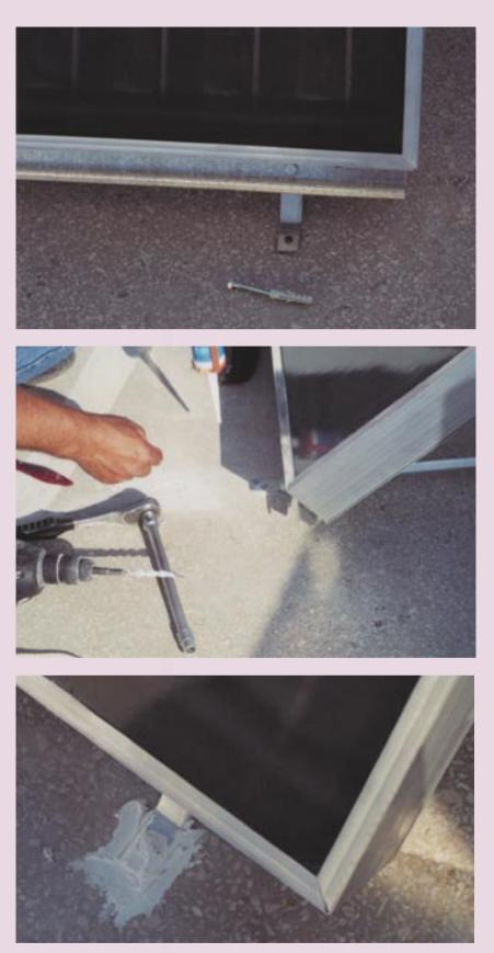
Figure 4.15 Steps for fastening the mounting frame on a flat roof and water proofing of the relevant point
