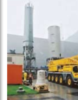
Closed cylindrical silo for animal meal storage. Source: STAG GmbH
