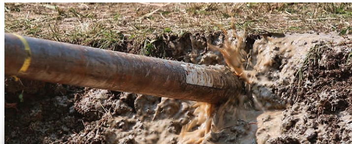
► ORFEUS HDD radar drilling during the field trials
