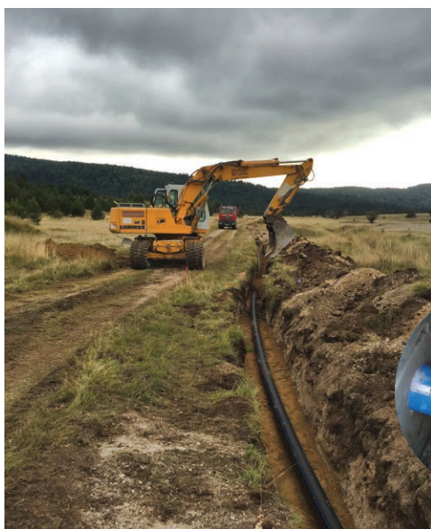
Construction of transmission-distribution main from the new Vrščić reservoir to the existing main city reservoir Gradina (HEIS, 2015)
