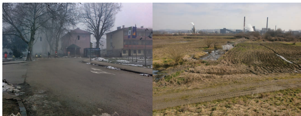
Lukavac WWTP site (NAMA, 2015)
