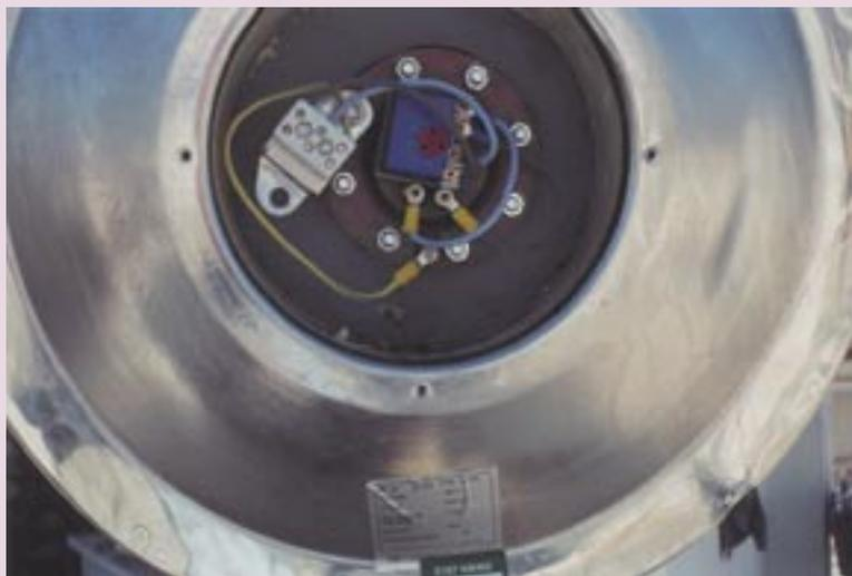
**Figure 4.16 Flange side of the hot water storage tank with the electric heater, the thermostat and the anode**
