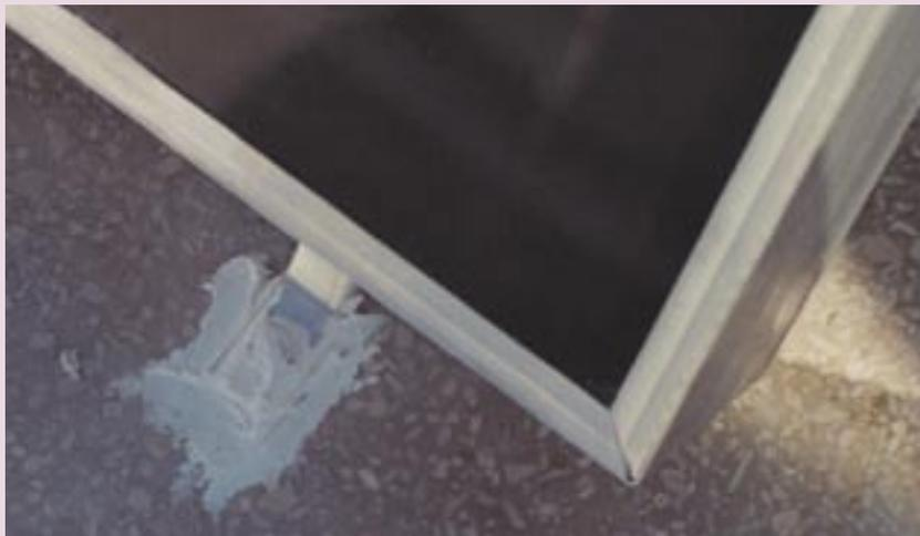
**Figure 4.15 Steps for fastening the mounting frame on a flat roof and water proofing of the relevant point**
